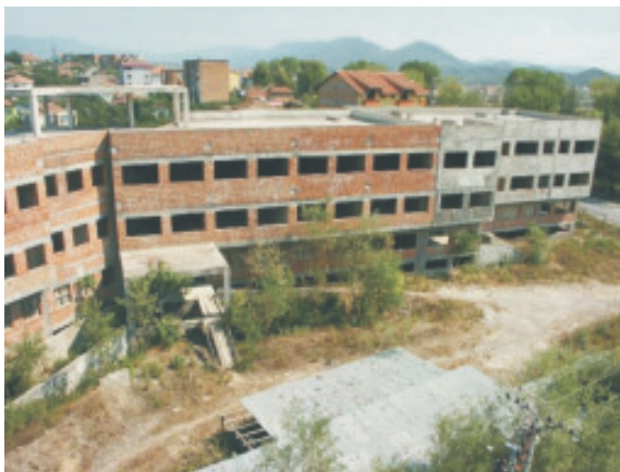
Al-Rahma Hospital Construction top view
