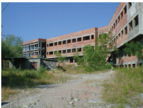
Al-Rahma Hospital Construction front view
